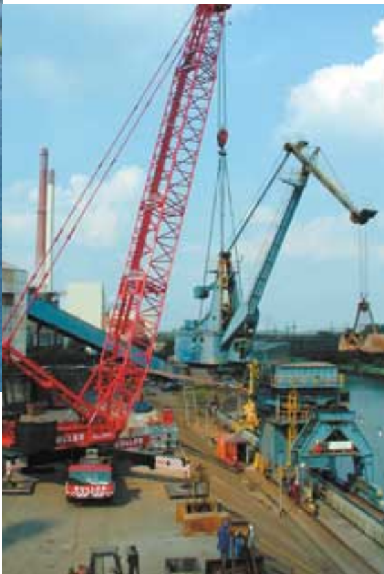
Repair/Replacement of the slewing bearing of a portal crane
