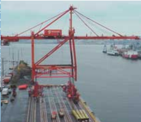
Upgrading two cranes by heightening the cranes by 6 meters
